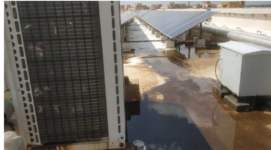
Image 6: Leakages in chiller supply and return water lines
